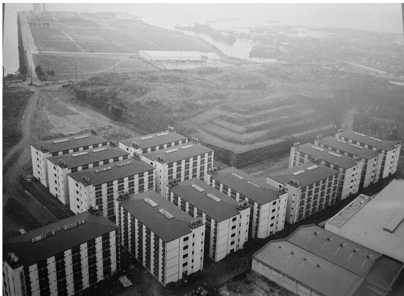
Fig. 2 – Paradise Heights during its construction. In order to realize the buildings, part of the dump-site was dug out and cleared. The rest of the heap was covered with land. (© Neil Oshima)
